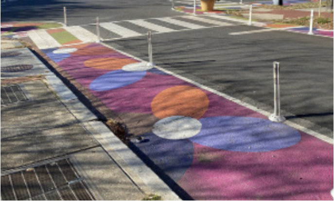
Artful Curb Extension / Removal of Parking
