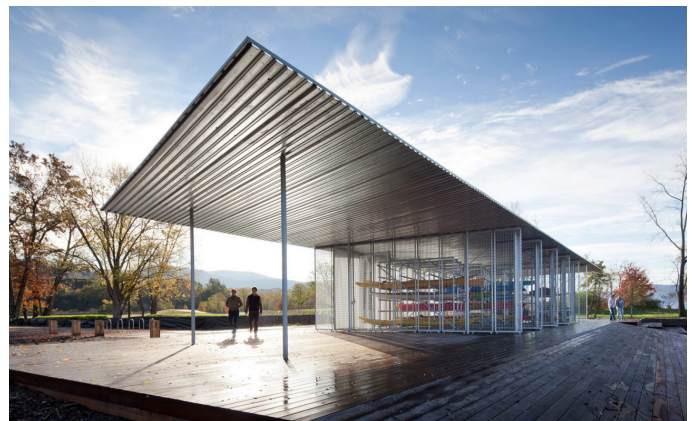
Boat pavilion and storage. Beacon, NY
