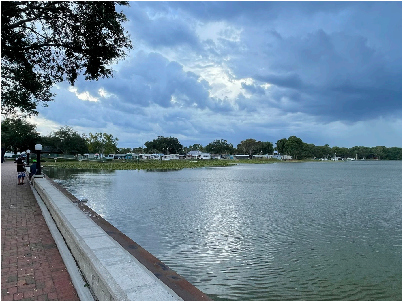
Existing Walkway at Ferran Park
